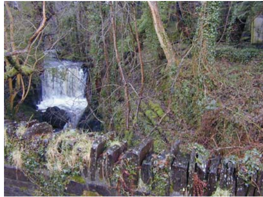
Old dam where tailrace must discharge
