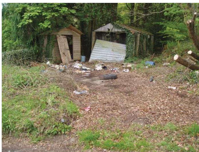
Existing structures at proposed powerhouse location
