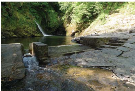
600l/s Perforated sheet installation
