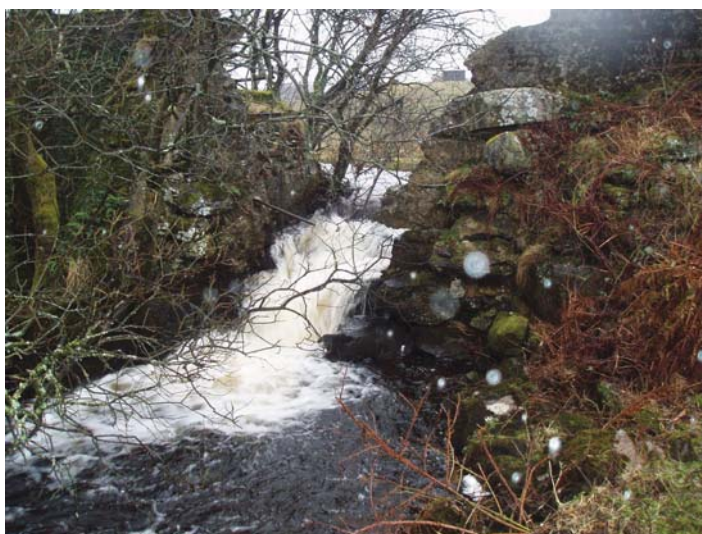
Remains of old dam for Galedffrwd scheme intake
