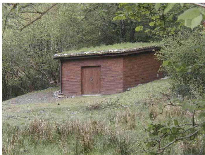
200kW Pelton turbine powerhouse
